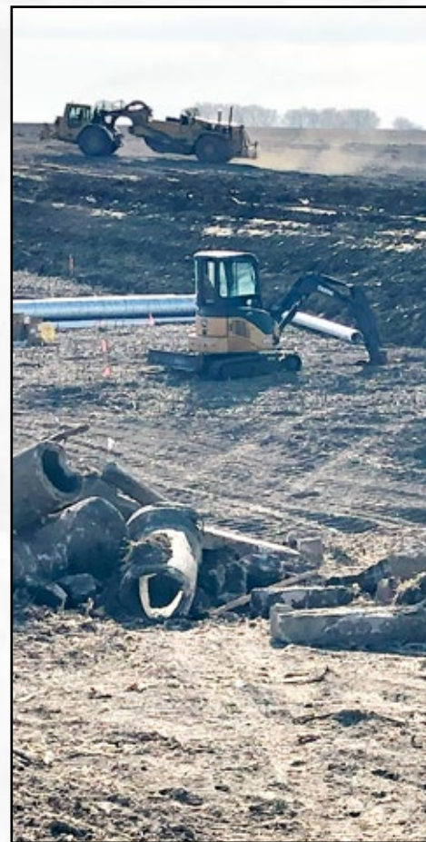
Heitmann Dam Construction in Mid March 2024.
