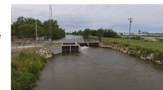
The renovated canals allow excess flows to be diverted and retimed.
