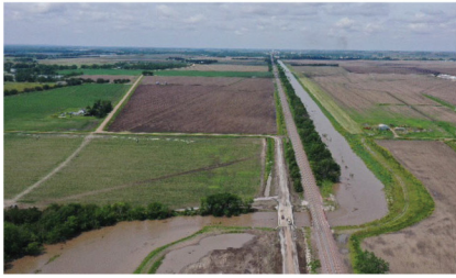
Aerial view of the Shell Creek and Union Pacific bridges rebuilt in 2021 during the recent heavy rains.
