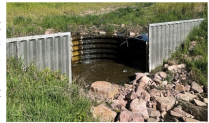
Completed drainage project in the Shell Creek Watershed
