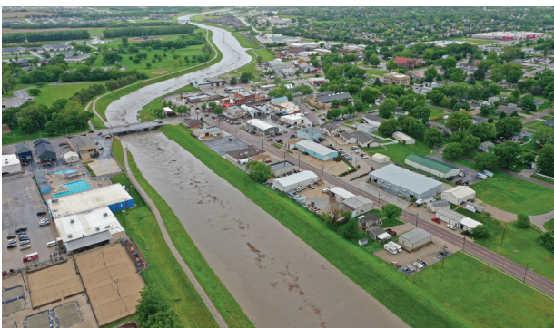
In the Papio-Missouri River NRD, floodwaters are channeled down the Papio Creek to nearby storage reservoirs in the Omaha metro preventing flooding during a heavy rain event in spring 2024.
