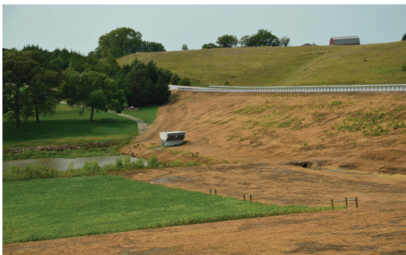
Lower Platte South NRD rehabilitated Upper Salt 3-A near Sprague, Nebraska. Originally constructed in 1955, the Upper Salt 3-A Dam was upgraded to meet high hazard standards and completed in fall 2021 at a cost of $1.9 million. The project included raising and widening the dam, expanding the auxiliary spillway, increasing flood pool storage, installing a new inlet structure, a larger principal spillway pipe, and a plunge pool impact basin to slow discharge flows. NRCS covered 65% of the funding through the Watershed Rehabilitation Program, with Lancaster County contributing by realigning the county road as part of the project.
