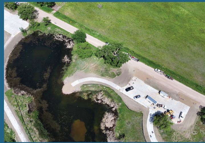
In February 2024, Central Platte NRD began renovations on the Alda Crane Viewing site near Alda, Nebraska. Renovations included a new viewing platform, paving the recreational trail and two parking lots to make the area fully ADA accessible. Other improvements included angler access to the pond and bank stabilization.
