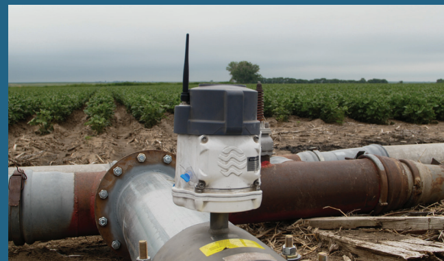
All irrigators in the Middle Republican NRD are now equipped with telemetry meters to improve irrigation efficiency.
