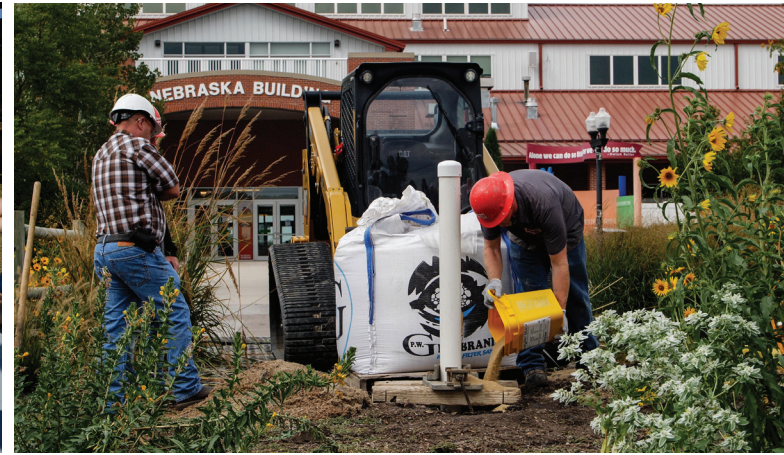
The public can now explore groundwater levels at the Nebraska State Fairgrounds. A recent addition to the site is a monitoring well, installed by the Nebraska Well Drillers Association and built by Downey Drilling, which reaches a depth of 55 feet. Seim Ag Technology donated a sophisticated monitoring system to provide real-time data on groundwater levels. Central Platte NRD will monitor this well, which has been added to its 116 active monitoring wells from Gothenburg to Columbus. Data collected from these wells, along with 500 irrigation wells, is vital for the NRD's groundwater management program, with measurements taken each spring and fall.
