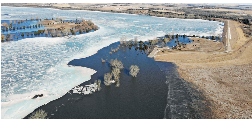
Willow Creek State Recreation Area, southwest of Pierce in the Lower Elkhorn NRD, held back more than 18,000 acre-feet of water during the historic March floods totaling more than 5.86 billion gallons of water.
