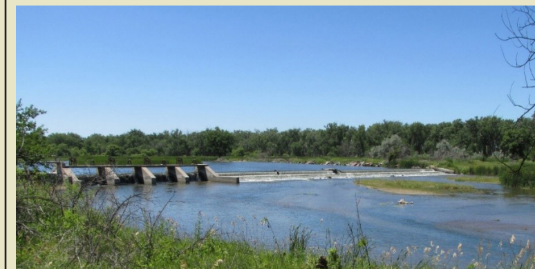
Finished Pipeline, Twin Platte NRD
