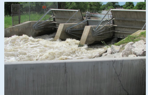
Basin Tour 2015 - Central Platte NRD Canals
