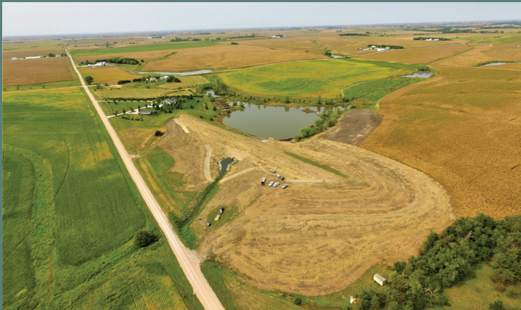
Lower Big Blue NRD nears completion on Little Indian 15-A, north of Pickrell. The project included adding a second emergency spillway, raising the height of the dam and installing a new tube.
