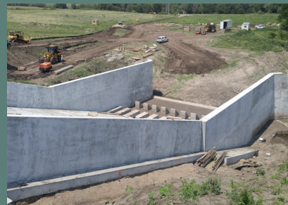
Above: In December 2020, work was completed on the Upper Big Nemaha 25C dam concrete spillway.
