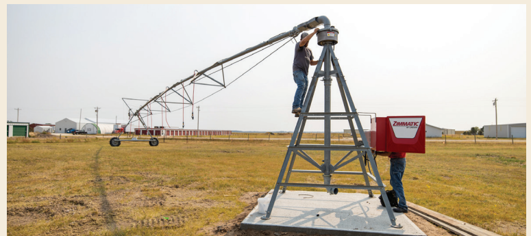
Lindsay Corporation donated a 121-foot center pivot irrigation system for Middle Niobrara NRD's outdoor training center. The pivot will be set up with a chemigation system, flow meter, and technology control panels to provide hands-on training for groundwater technicians across the state.
