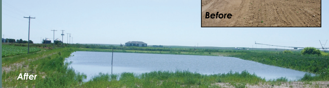
In Deuel County, South Platte NRD is using a reuse pit recharge program to manage South Platte River excess flows for groundwater recharge, mitigating downstream flooding and improving stream depletions.
