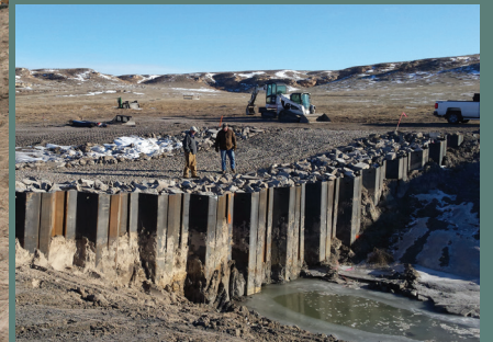
Upper Republican NRD installed the Rock Creek drop structure near Parks to reduce channel erosion due to water releases from the Rock Creek augmentation project.
