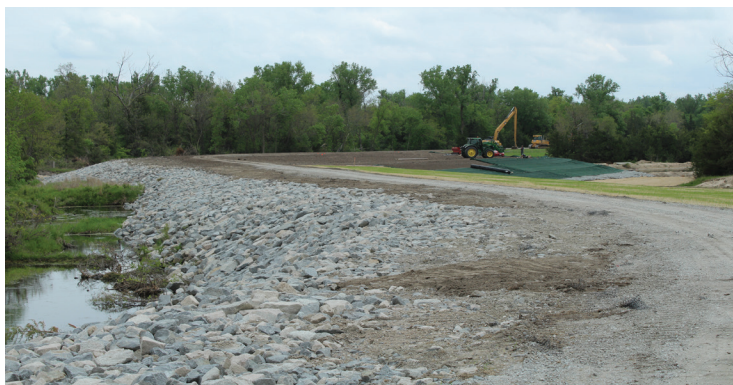
Lower Platte North NRD makes repairs on Clear Creek in May, which was breached during the 2019 flood.
